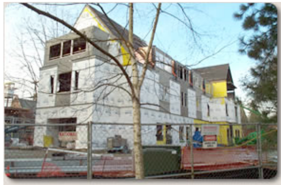
The ETC, under construction
